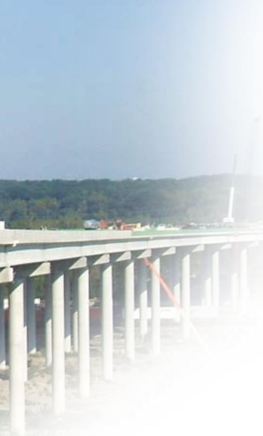
JSE created this option along with a steel-plate girder alternative, using two design teams that each presented their approach to the contractor, Walsh Construction Group in Chicago. "Walsh did the calculations and added up all the costs and chose the concrete design," Spaans says. "They made the choice based on the bottom line."
