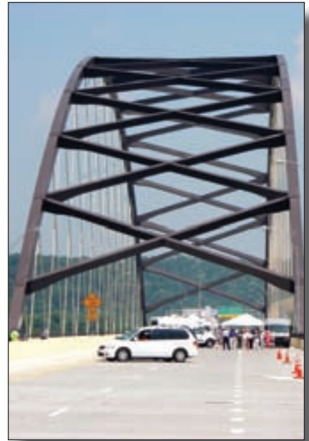
"The Blennerhassett Island Bridge is a signature structure designed by engineers who were willing to test the limits of traditional engineering methodology."
