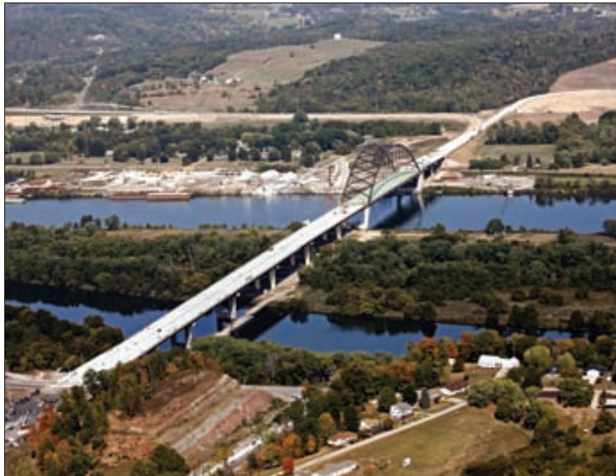
The total length of the Blennerhassett Island Bridge is 4,008 ft from abutment to abutment. The structure includes an 878-ft-long tied-arch main span whose apex towers 245 ft above the Ohio River.
