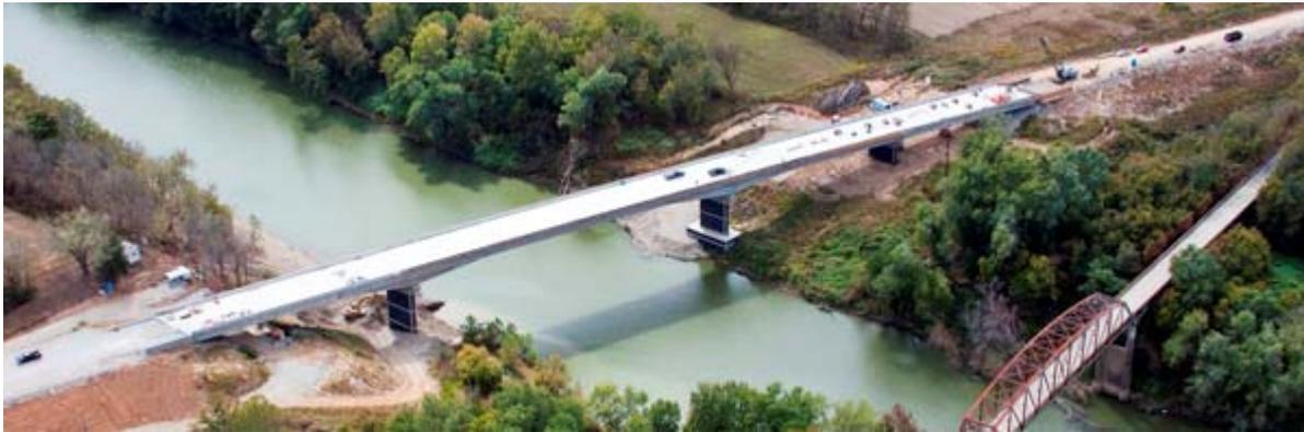
**High strength concrete was used for the precast, prestressed concrete beams.**
