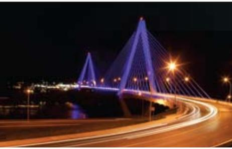
*The Bridge of Honor, also known as the Pomeroy Mason Bridge, is a concrete cable-stayed bridge with a 675 foot main span crossing the Ohio River. This bridge replaces a functionally and structurally deficient truss bridge connecting the towns of Pomeroy, Ohio with Mason, West Virginia, and provides a vital link between these two communities.*
