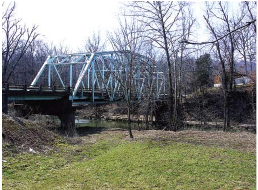
Old, deteriorated, steel-beam truss bridge over the Little Scioto River.
