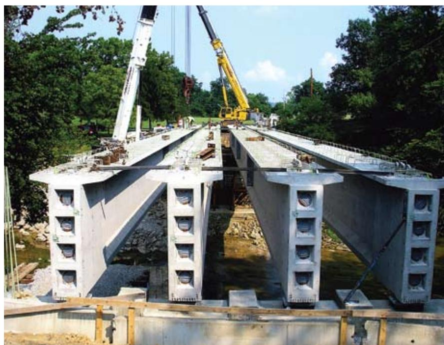
Newly installed, precast concrete bulb-tee girders.
