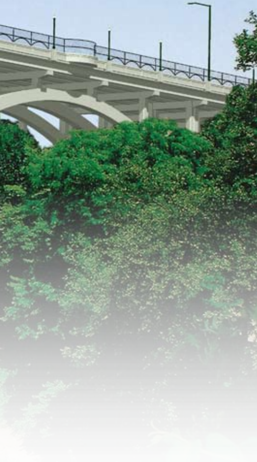
A rendering showing the Fulton Road Bridge traversing the Big Creek Valley and a walkway at the Cleveland Metroparks Zoo. Illustration: Michael Baker Jr. Inc.
