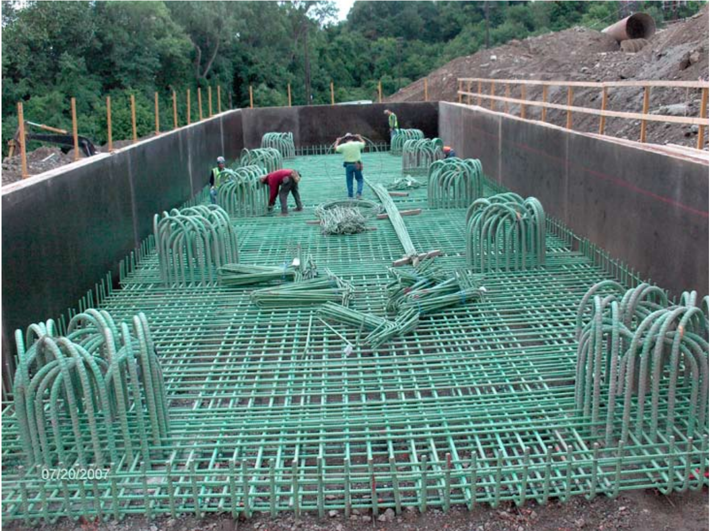
Reinforcement in the footing on 6-ft-diameter drilled shafts. Photo: Ohio Department of Transportation.
