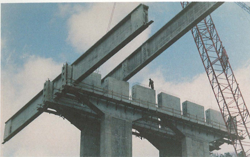
Fig. 4. Pier segments fit in pier cap slots.
