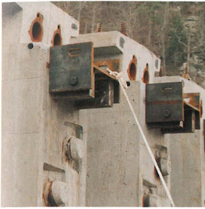
Fig. 18. Cazaly hangers in pier segment end blocks are ready to support drop-in segments.
