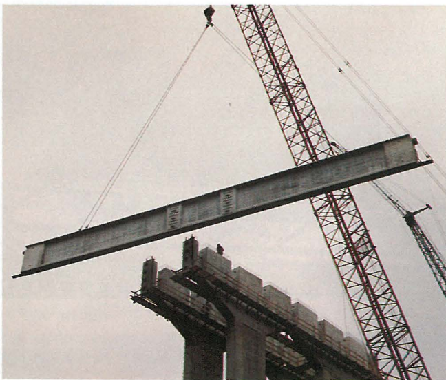
Fig. 16. Hoisting of 108 ft (33 m) bridge beam.
