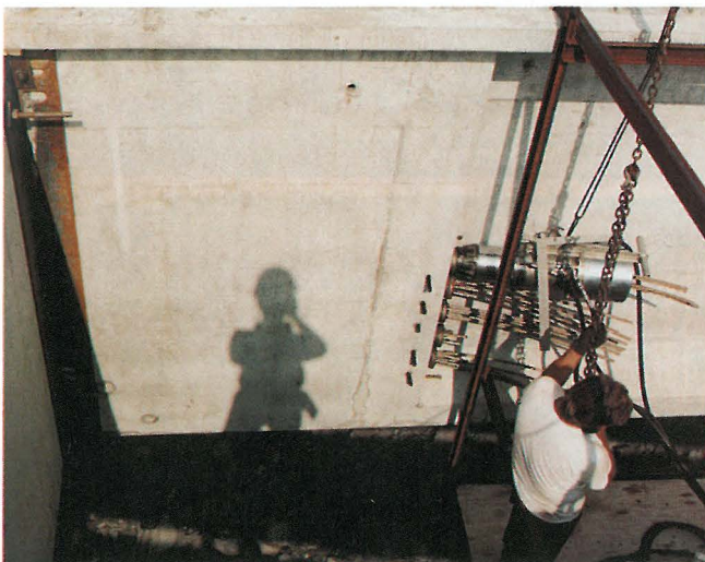
Fig. 20. Post-tensioning the splice tendons through beam end blocks.
