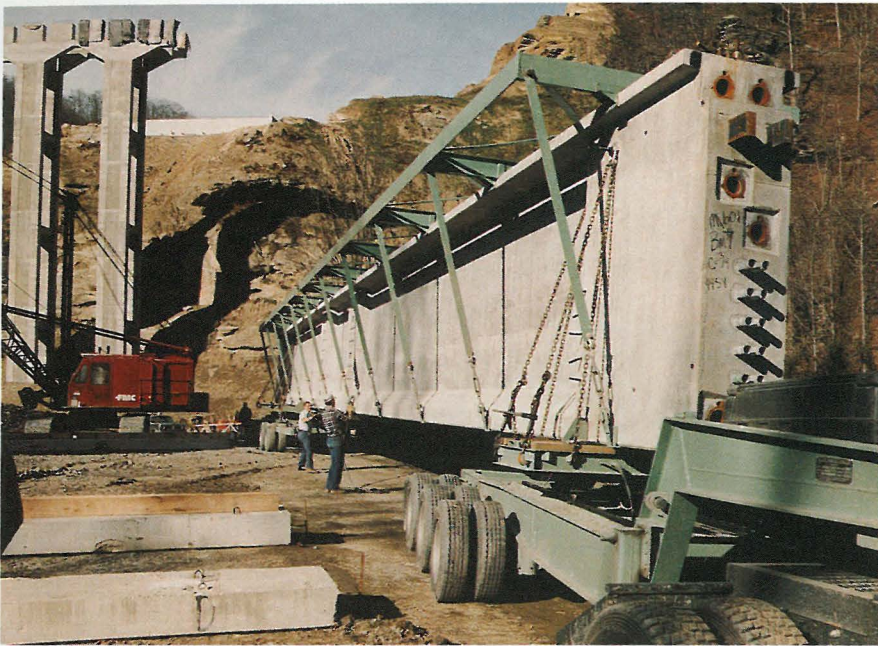
Fig. 14. Special trailer and stabilizing frame used to haul 108 ft (33 m) bridge beams.
