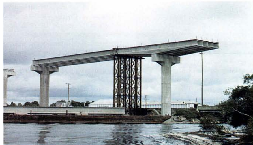
Fig. 12. Completion of span adjacent to main span.
