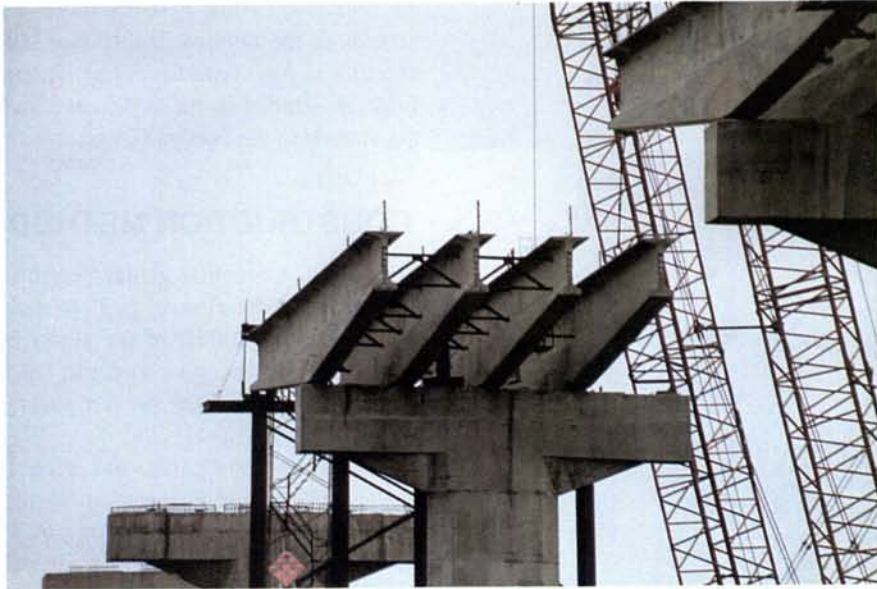
Fig. 10. Installation of haunched girder sections over piers.
