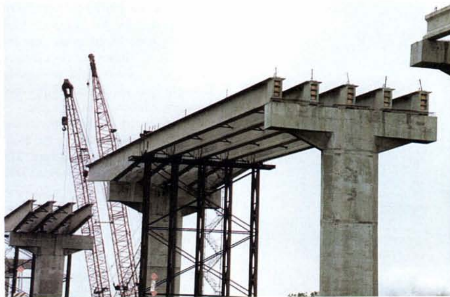
Fig. 11. Erection of end spans over piers.
