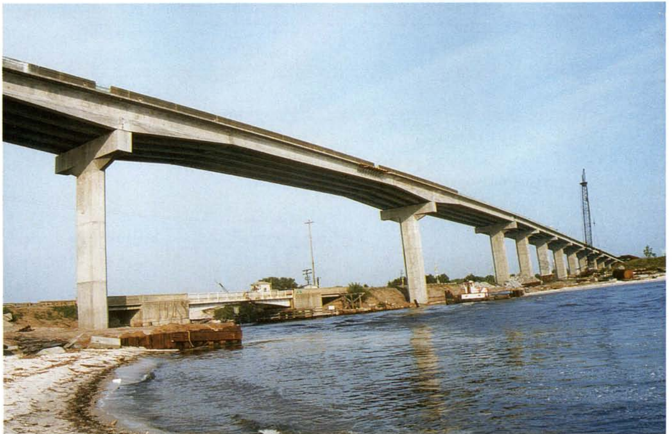
Fig. 2. Partial view of Highland View Bridge showing 250 ft (76.2 m) main span in foreground.
