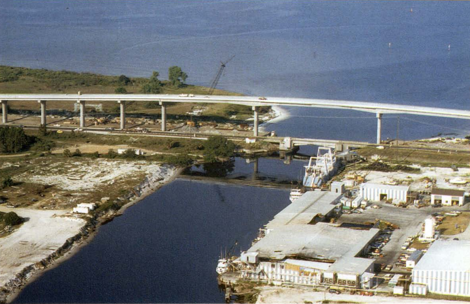
Fig. 1. Aerial view of Highland View Bridge showing record-setting main span.
