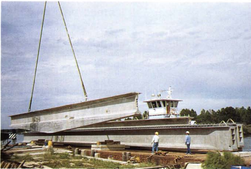
Fig. 9. After arrival at the bridge site, a haunched girder section is lowered by crane for temporary storage.
