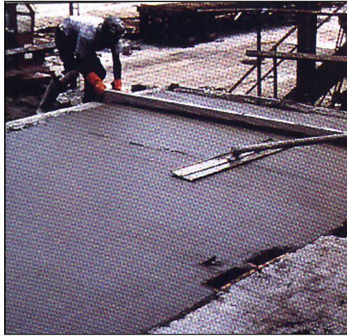
Figure 2. A high-quality finish of the top surface is essential in superstructure segments where it is also the riding surface.
