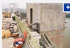
Bracket to hold the force regulating units.
