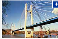
The Maysville Bridge is also known as the William H Harsha Bridge.
