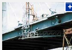
The Maysville Bridge, which carries US Highway 62/68, was completed in 2000.
