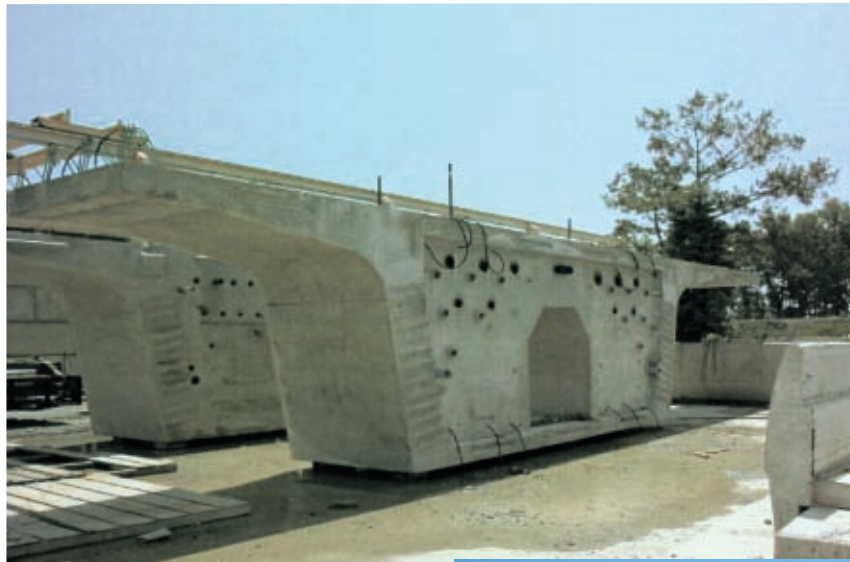
Figure 15 - Pier segments, New Victory Bridge, New Jersey
