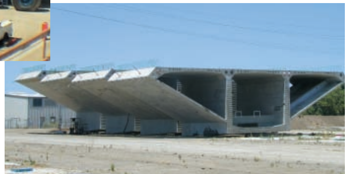
Figure 4 - Segment storage, San Francisco-Oakland Skyway Bridge
