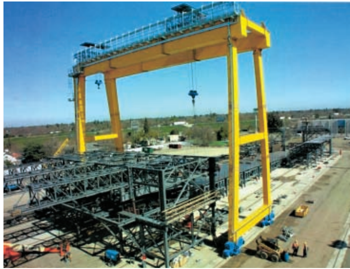
Figure 1 - Gantry at long-line casting bed 2F, San Francisco-Oakland Skyway Bridge
