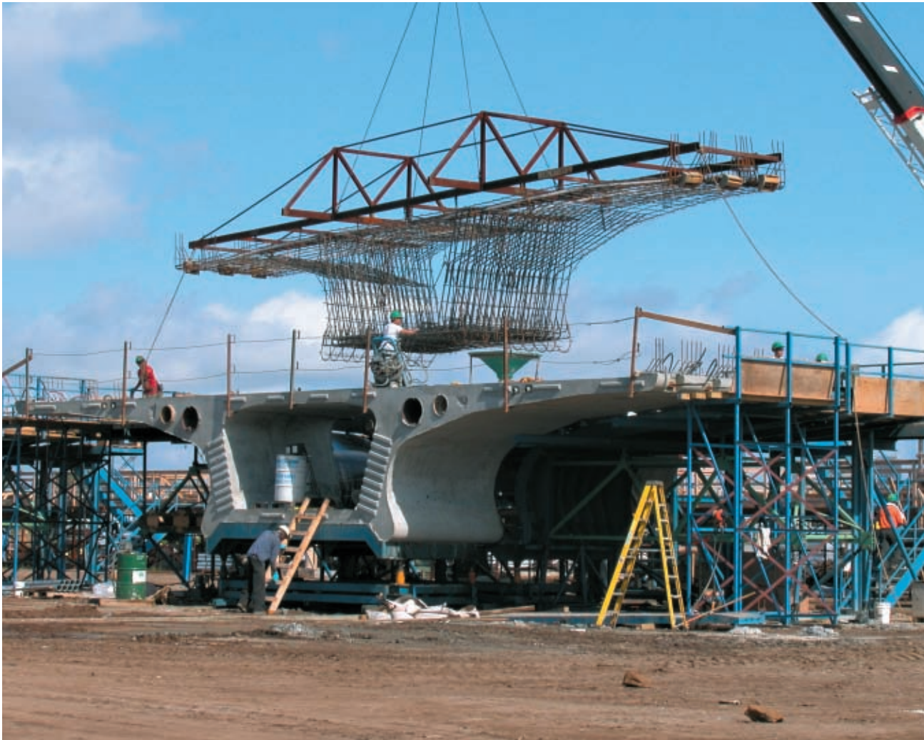
Figure 10 - Casting operations, Lee Roy Selmon Crosstown Expressway expansion, Tampa, Florida
