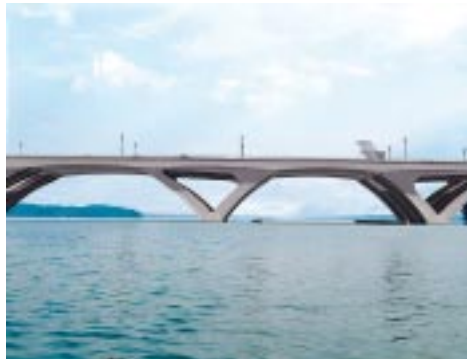
New Look. V-shaped concrete piers mimic upstream Memorial Bridge's arches.
