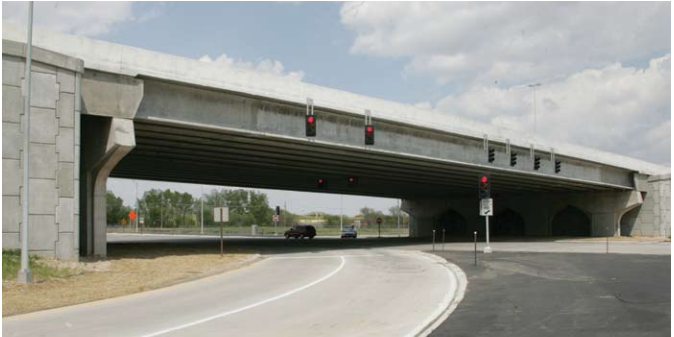
Fig. 1. A view of the 204th Street Bridge in Douglas County, Neb.
