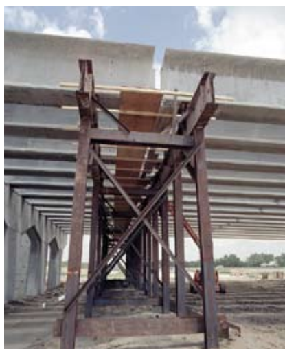
Fig. 9. A close view of a temporary tower and segment joint.
