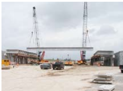
Fig. 7. Center segment prior to placement over temporary towers.
