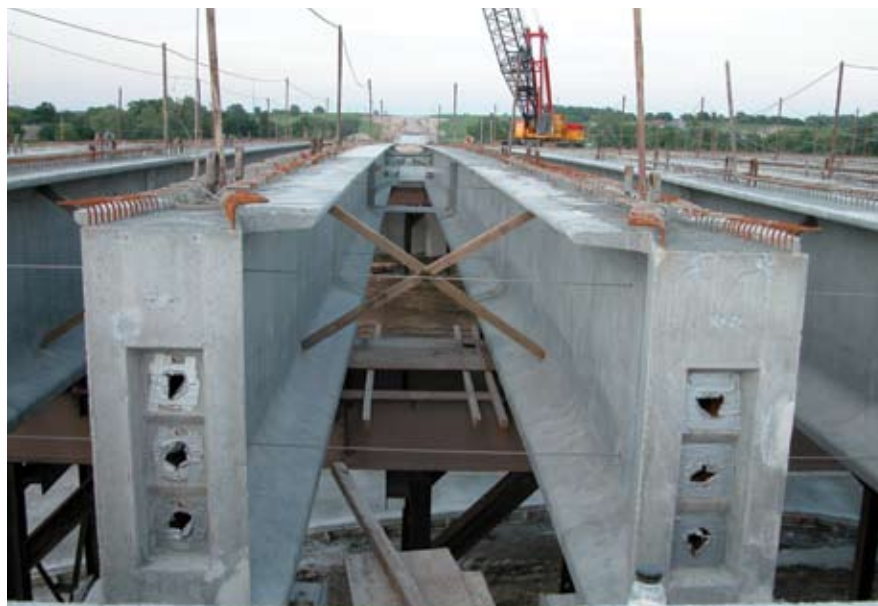
Fig. 6. Optimized post-tensioning end block.
