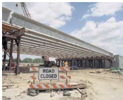
Fig. 8. All girder segments placed over piers and temporary towers.
