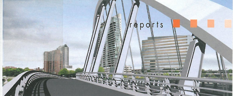
The bridge must be compatible with its neighbour Right: View along the structure
