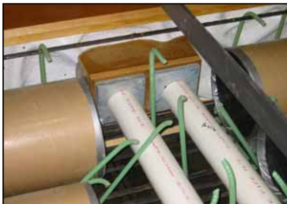
Inside a prestressed voided slab.
