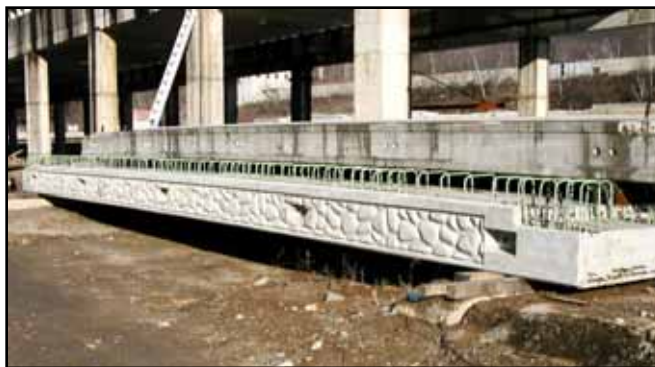
Exterior beams cast with a cobblestone finish.
