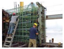
End girder detail prior to placing concrete in the girder.
