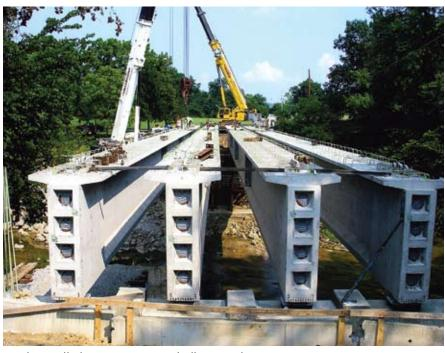
Newly installed, precast concrete bulb-tee girders.
