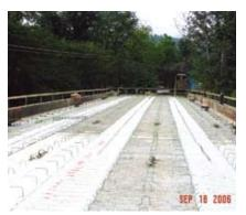
Bridge surface ready for 8½-in.-thick (216 mm) deck slab.
