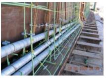
Swept ducts in girders prior to concrete placement.
