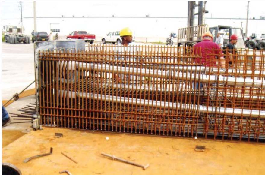
Fig. 16. Girder reinforcement, elevation view.
