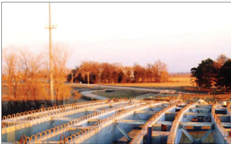
Fig. 20. Installation of intermediate steel diaphragms.
