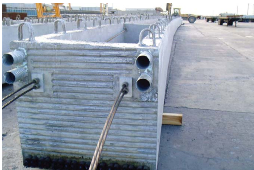
Fig. 17. Precast concrete girder stored in the precasting yard.
