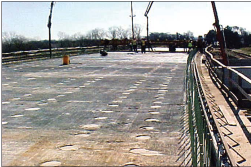
Fig. 23. Placement of overlay concrete.
