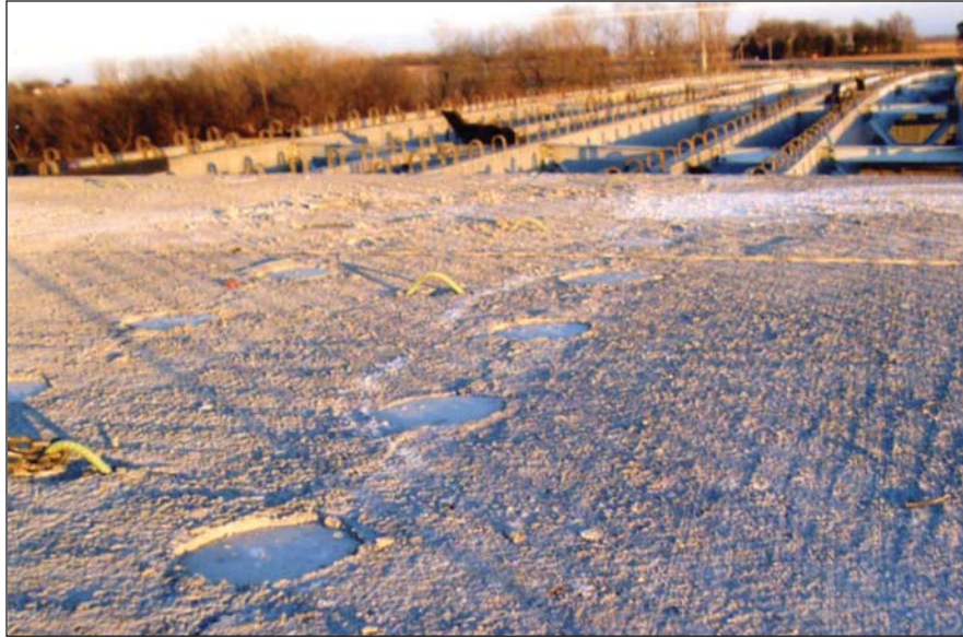
Fig. 22. Precast concrete panel installation.
