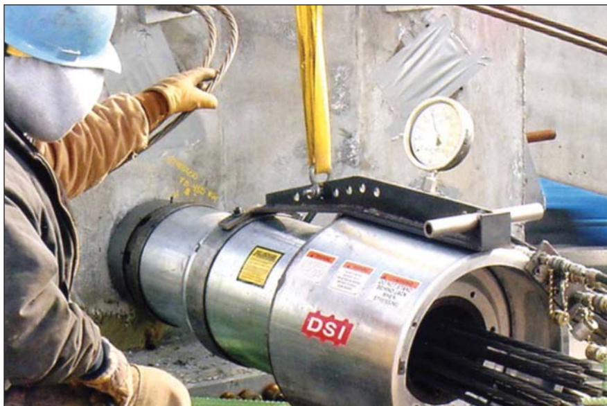
Fig. 21. Post-tensioning lower tendons.
