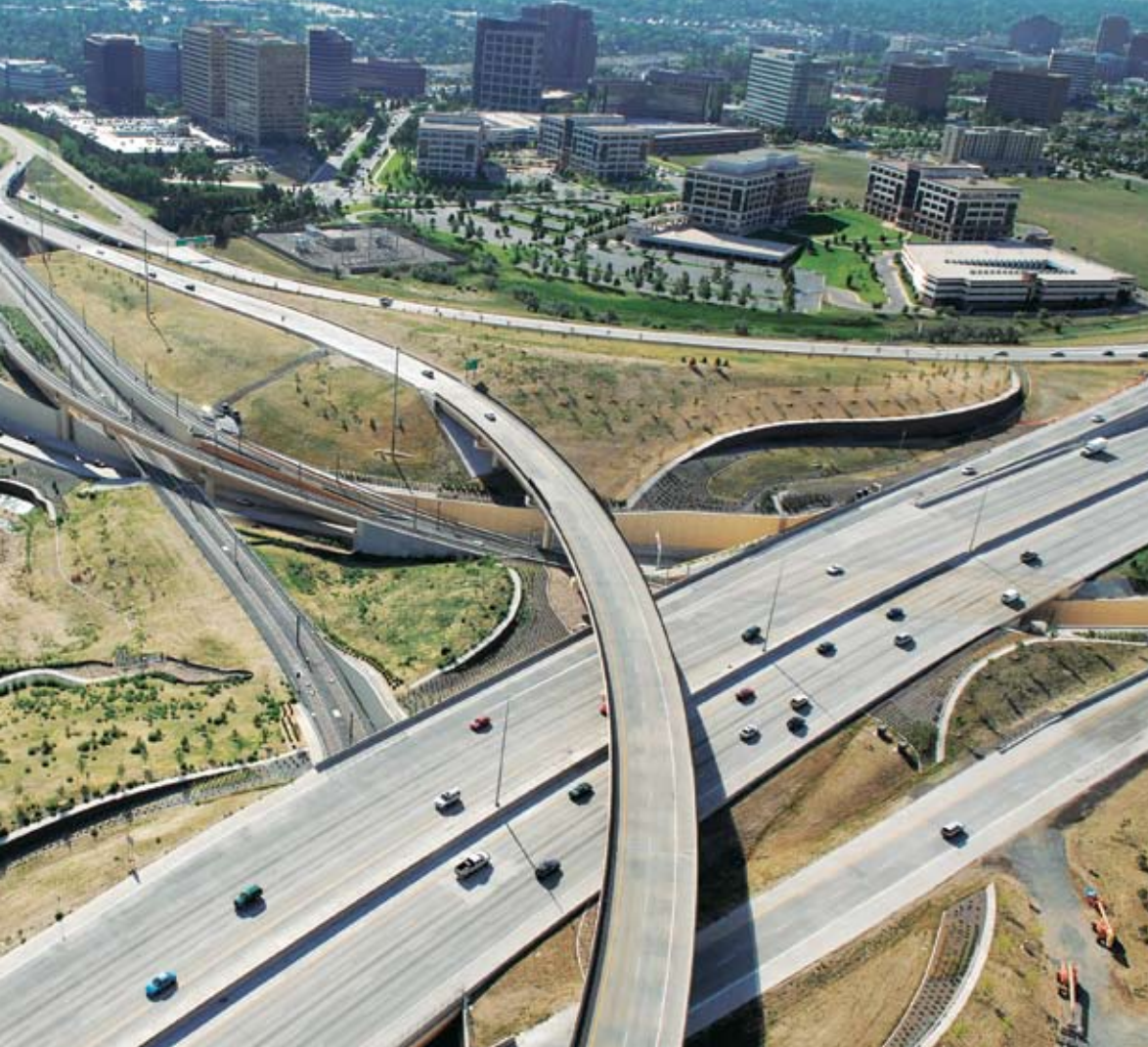
Designers on the Southeast Corridor Transportation Expansion Project (T-REX), the largest transportation contract in Colorado history, reconfigured the interchange to move light-rail trains from the highest level to the lowest. The changes resulted in significant cost savings, aesthetic improvements, and enhanced temporary traffic control. Photo: Parsons and Colorado Department of Transportation.
