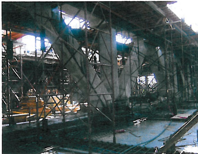
Fig. 5: View of the center of a nearly complete transfer truss
