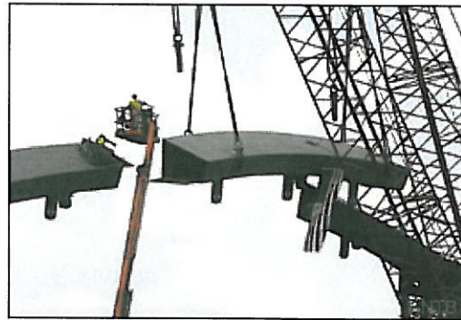
The center piece of Columbus bridge's arch is set in place.
