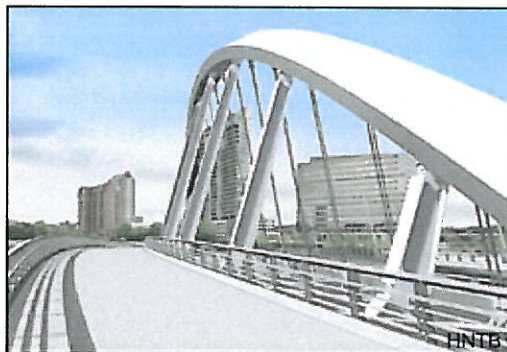
Arch is tilted 10° and tied with cable stays, with floor beams carrying walkway.
