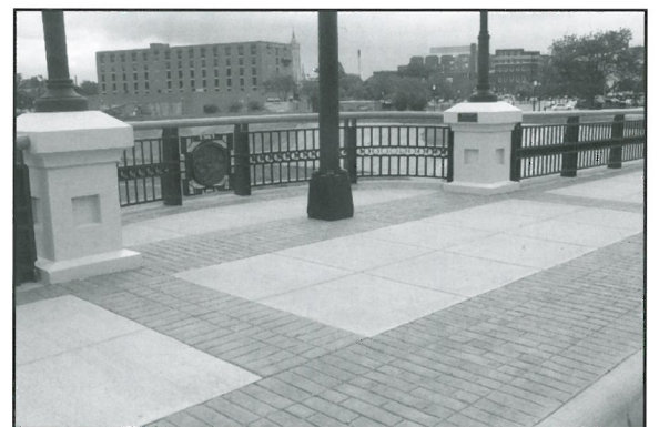
High attention to aesthetics was employed on both horizontal and vertical concrete surfaces on High-Main Street Bridge
