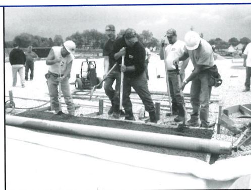
Hayslett Construction crew train on various pervious concrete placement steps
