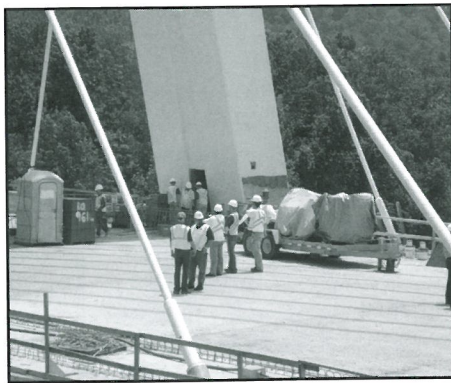
Tour attendees on the deck to witness the scale of the structure first-hand
