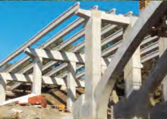
All photos: Ohio Department of Transportation.
