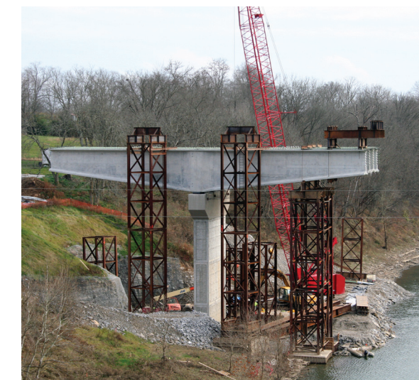
Temporary towers supported steel beams spanning over the piers that in turn supported a gantry with strand jacks to lift the pier segments and move them laterally into place. Photo: Haydon Bridge Co.
