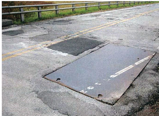
Bridge over Grassy Creek: Steel plate over deck deterioration.
