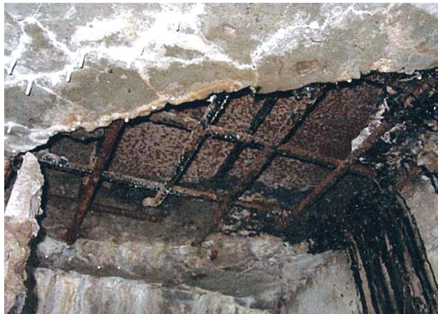
Bridge over Grassy Creek: Severe deck deterioration at west end.
