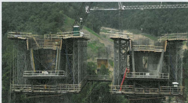
This complex twin-segmental box bridge will reach over 1,700 ft in length and reach a height of 250 ft. The bridge includes 15,340 sq ft of pre-assembled Top 50 formwork that builds four sets of traveler forms.
