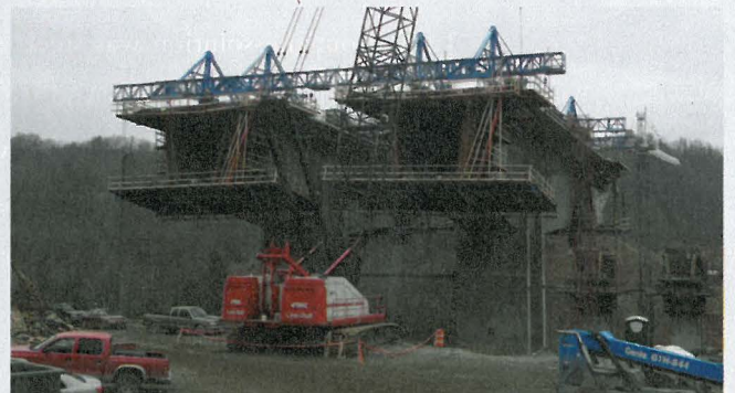
This complex twin-segmental box bridge will reach over 1,700 ft in length and reach a height of 250 ft. The bridge includes 15,340 sq ft of pre-assembled Top 50 formwork that builds four sets of traveler forms.
