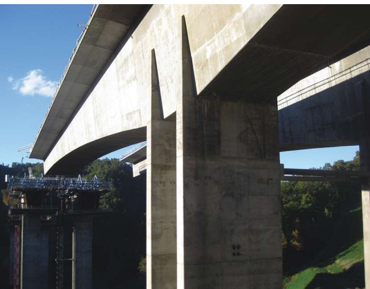
The walls of the H-shaped pier columns continue into the box girder to provide an integral connection.
