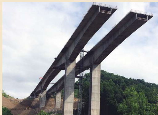
Two of the completed cantilevers highlight the curves of the structure.
