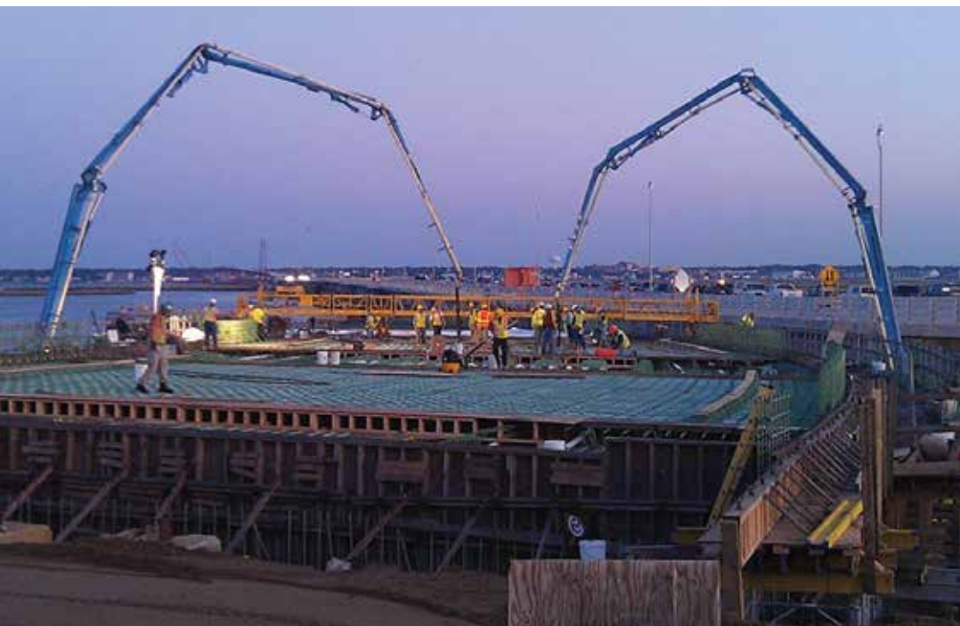
Fig. 1—Concrete placement on Route 52 Bridge.
