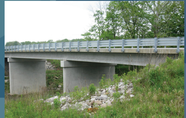
BRIDGE 25 OVER SAND CREEK JENNINGS COUNTY, INDIANA
